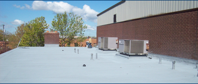
SPF Encapsulation Penetrations
