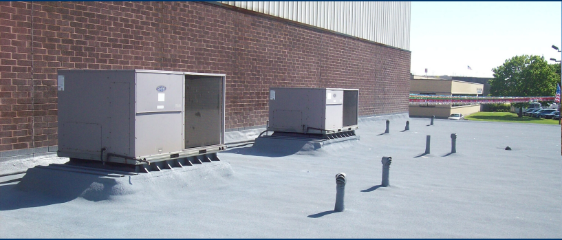
SPF Encapsulation Penetrations
