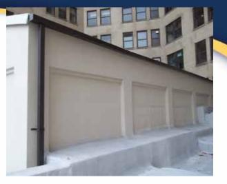
energy efficient, and cost-effective system available. Portions of this foam work, especially over the windows of the vertical auditorium walls, had to be installed to appear as though no work had been done to the original construction. The termination points, feathered edges, and overall smooth appearance of the application were absolutely critical to the success of the project.
